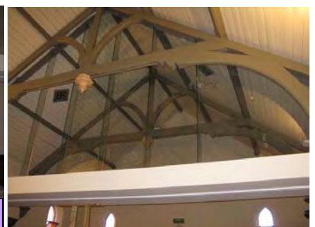
Glass above the Operable Wall
