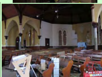
Worship Space - removal of pews and old flooring, installment of flooring & preparations for painting, installation of wiring for the two screens.
